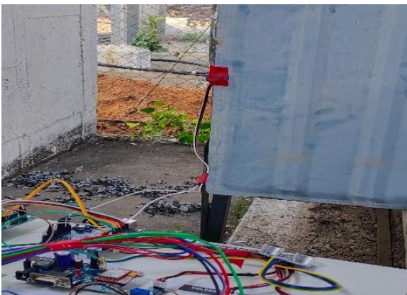
Figure 19 Radiator in Temperature Monitoring
