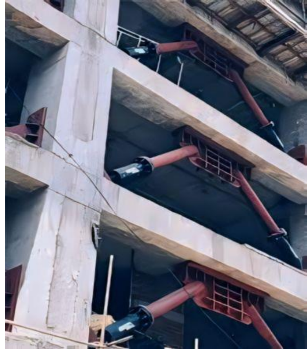
Figure 1 Viscous Damper
