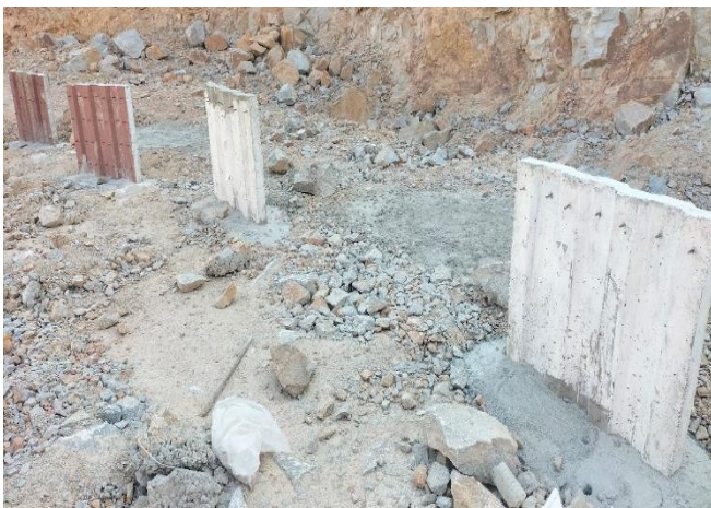
Figure 3 Experimental Set up of Composite Wall Panel
