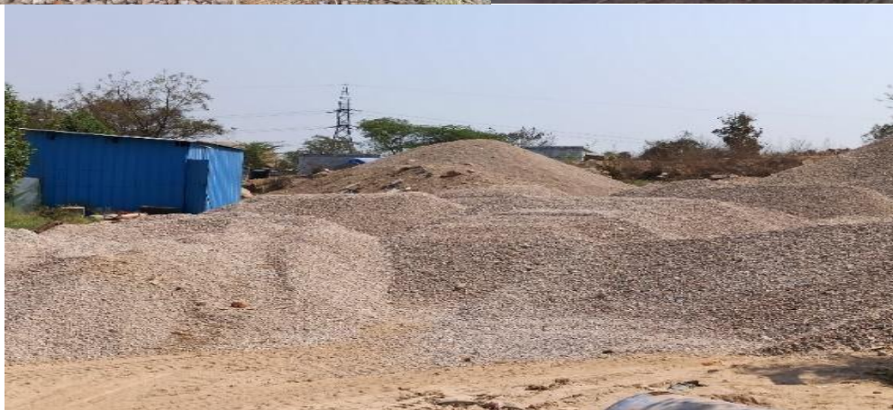
Figure 4 Sand & Aggregates Prepared from C&D Waste
