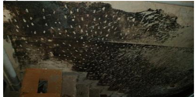
Figure 1 Soot Deposition in Building
