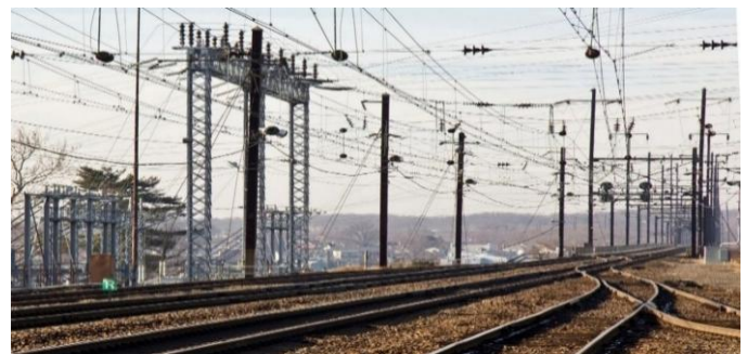
Figure 1 Flexible overhead catenary system
